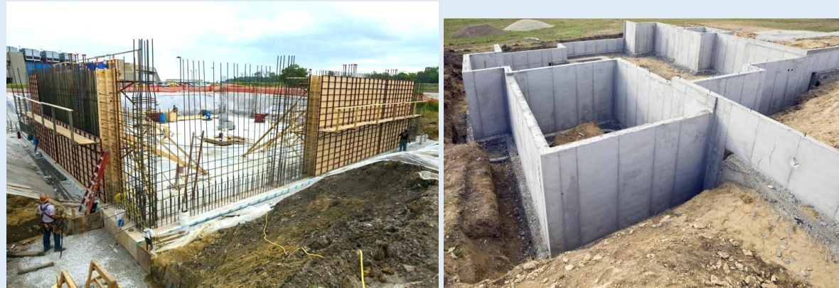
Foundations walls being built in a construction site
